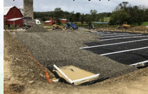
Subgrade with ridge-valley shape to expedite drainage
