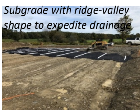
Subgrade with ridge-valley shape to expedite drainage
