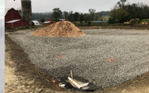
Ready for wood chip placement over stone
