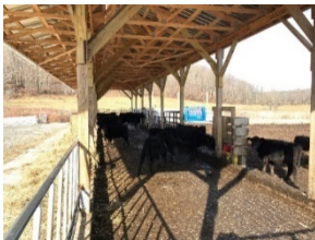
Concrete, covered feed lane adjacent to wood chip pad
