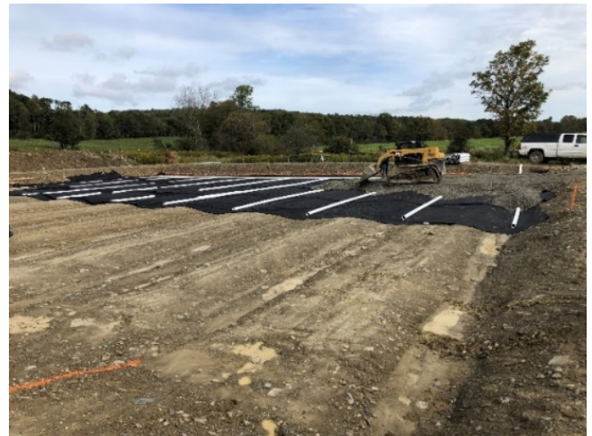
Subgrade shaped in ridge and valley pattern to expedite drainage.
