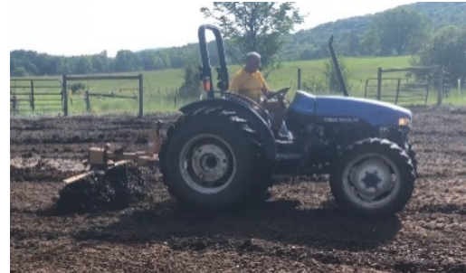
Six inches of soiled chips removed with back-blade.
