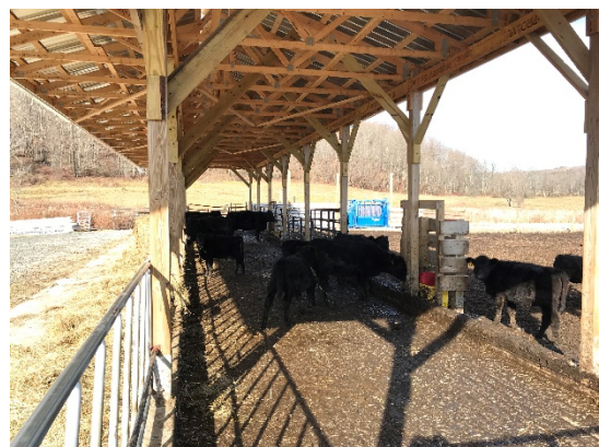
Concrete, covered feed lane adjacent to wood chip pad
