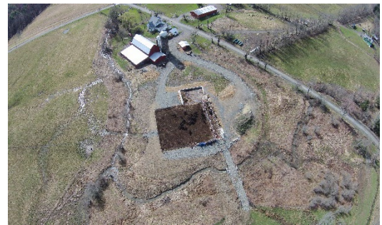
Aerial view of completed project (4/17/2019). Previous unimproved holding area was in the same location.
