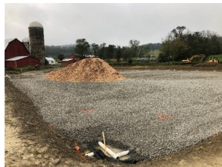
Ready to place wood chips atop #57 stone.
