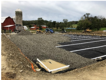
Clean #57 stone being placed over perf. pipe.
