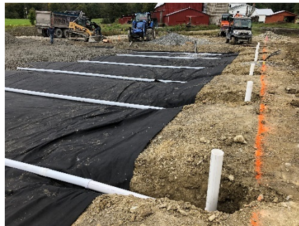
Clean-out at start of each perforated pipe.
