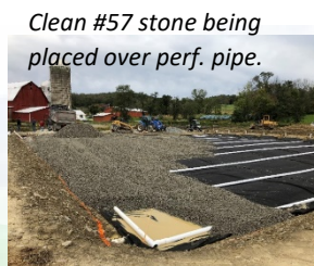
Ready for wood chip placement over stone
