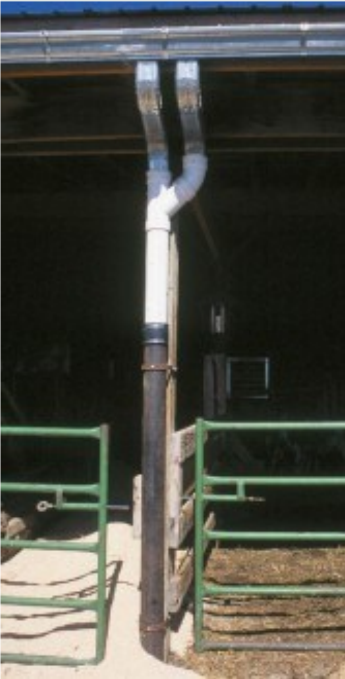
Roof Gutters to collect and divert water to a clean, stable outlet.
