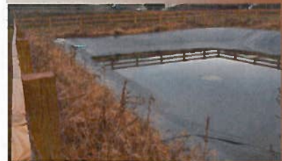
Drainage water holding pond constructed for effluent from a woodchip pad.
