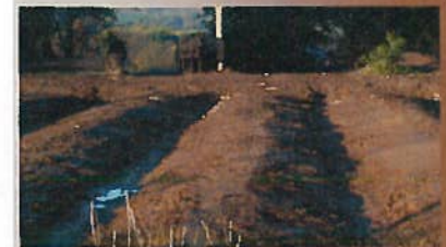
Shaping of woodchip pad subgrade to encourage drainage.
